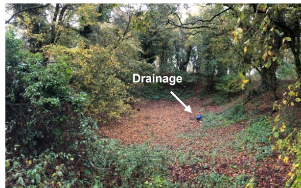
Photo 2 — Drainage Outfall in Hollow
